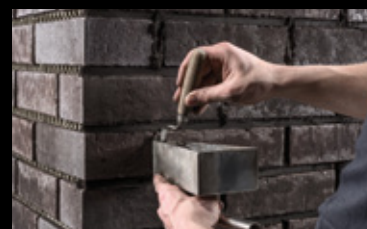
The vertical joints can be finished more easily with a smaller pointing trowel.
