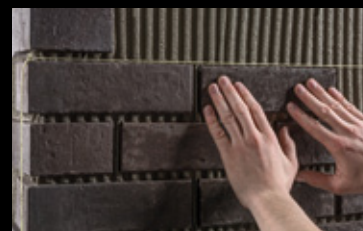
Use a string to plumb the clinker area. The clinker slips are pressed into the adhesive bed.
