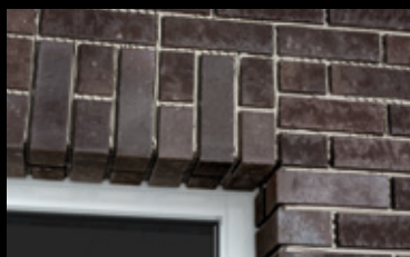
Window lintel perfectly replicated with angles.
